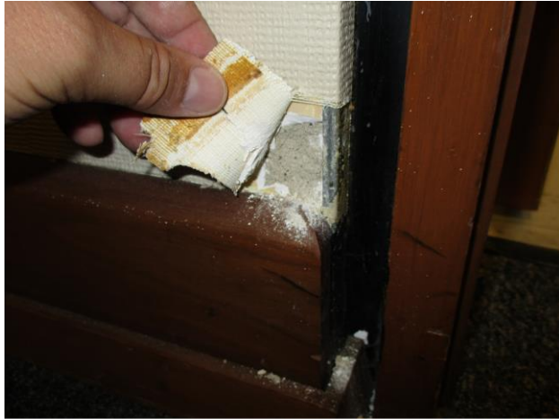
Non-ACM Wall Plaster
