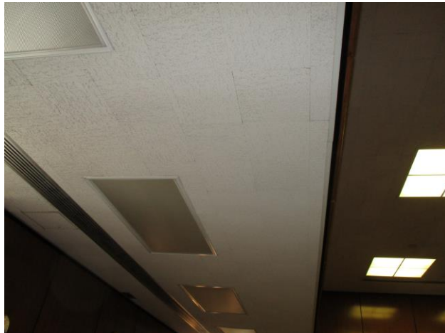
Non-ACM Ceiling Tiles
