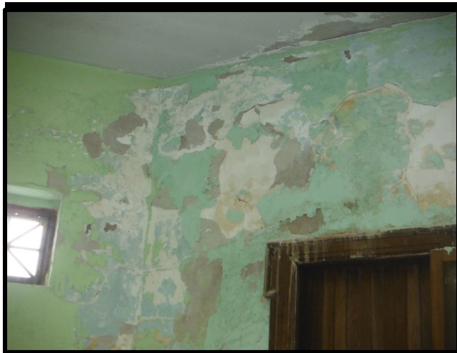
Water infiltration seeping through walls due to the breakdown of brick pointing, and poor roof conditions. This not only caused internal damage but mold as well.
