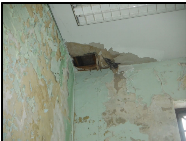
Internal ceiling damage from poor roof conditions (pitch and tar roof).
