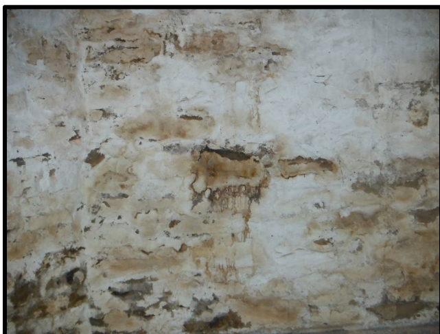
Field bricks allow water to seep into foundation which weakens structure and causes mold. Stairwell too steep and does not meet current codes or ADA compliance standards.
